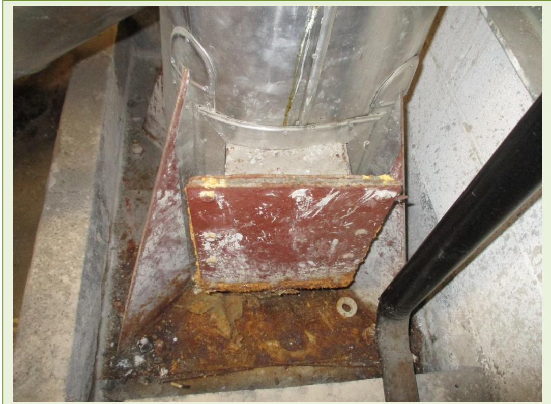
Rope between the ducting flanges in the 1 st floor plant room. No ACM's detected
