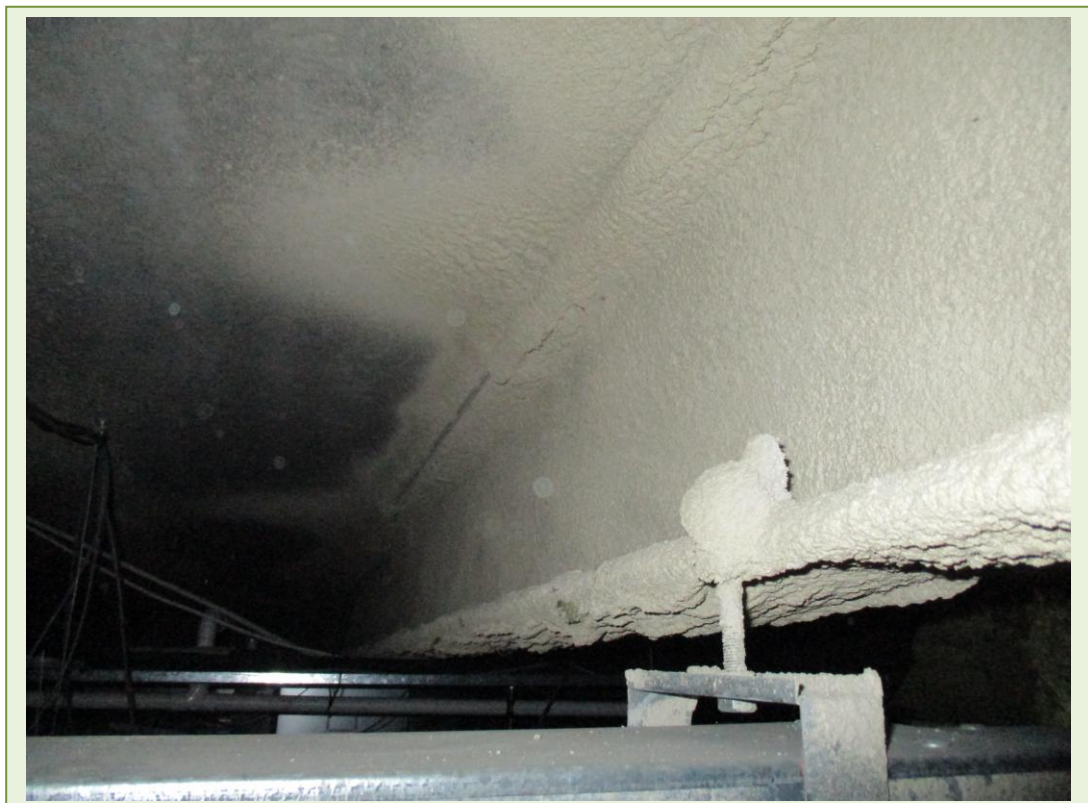
Sprayed coating on the beams in the office areas. No ACM's detected
